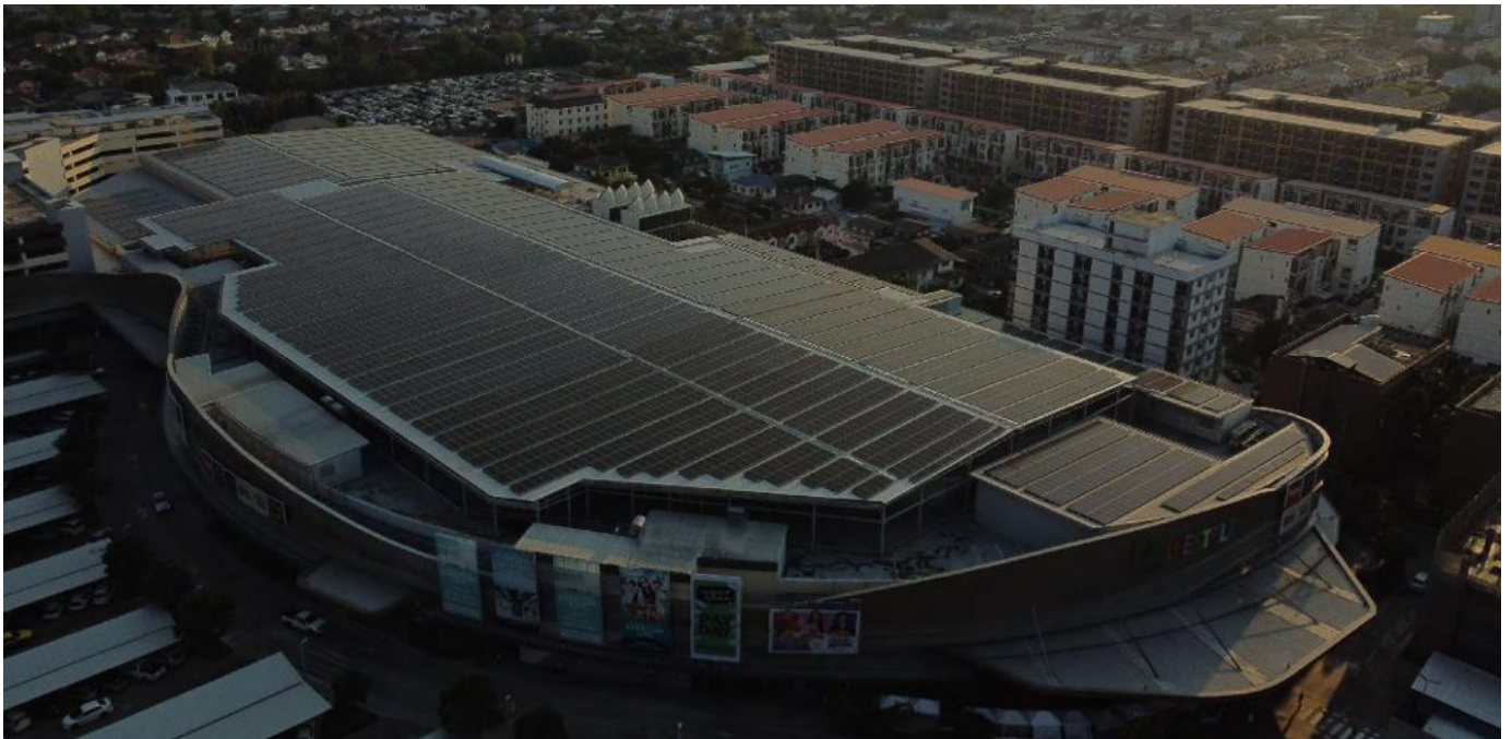
Robinson Ladkrabang - 4,129 kWp
